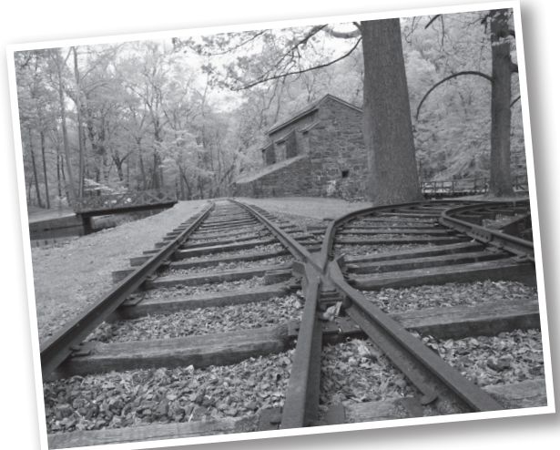
The Graining Mill in the Powder Yard at Hagley.
